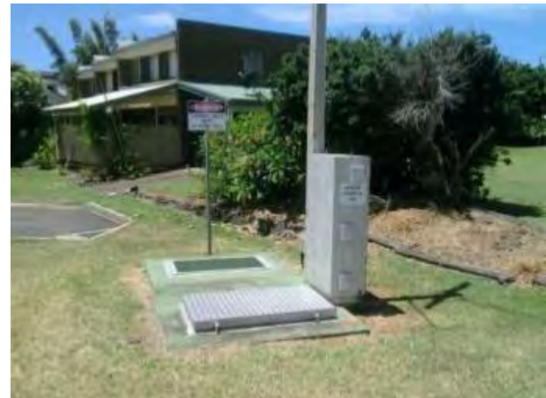
Typical SCADA controlled sewage system
