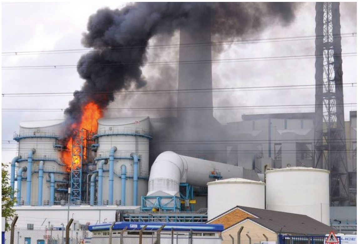
The Erebos Trojan causes critical damage to vulnerable generators, resulting in fire.
